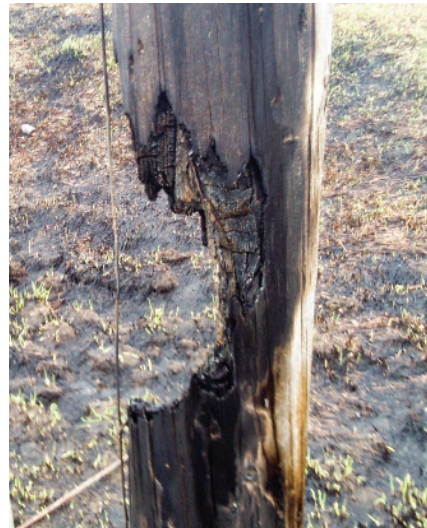
Before burning, check the property for electrical equipment and power poles to avoid damage and potential outages.
